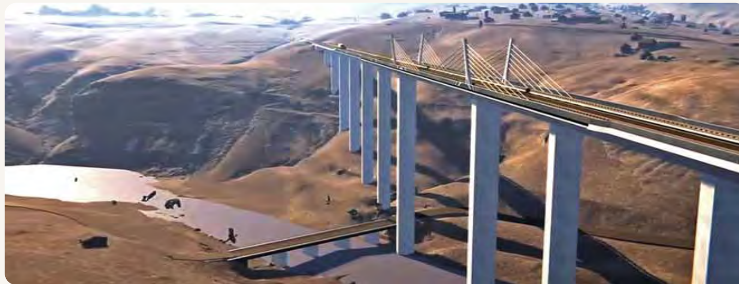
The artist impression of the main Senqu bridge poised to become the biggest bridge in Lesotho, at the height of 90 meters and length of 825 meters (copyright LHDA)
