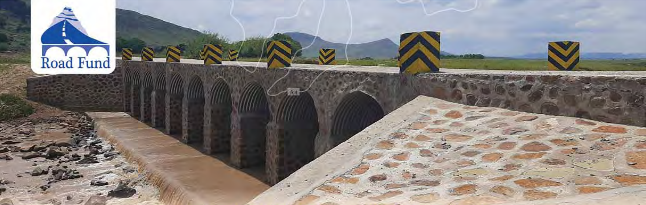
Routine Maintenance of Bongalla to Maseela road - Construction of a Vented Ford sponsored by Road Fund
